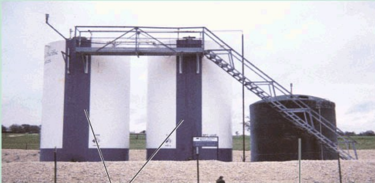
Oil/Condensate Tank
